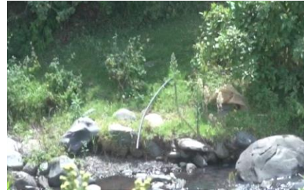
Figure 7: illegal pump (own photo)
