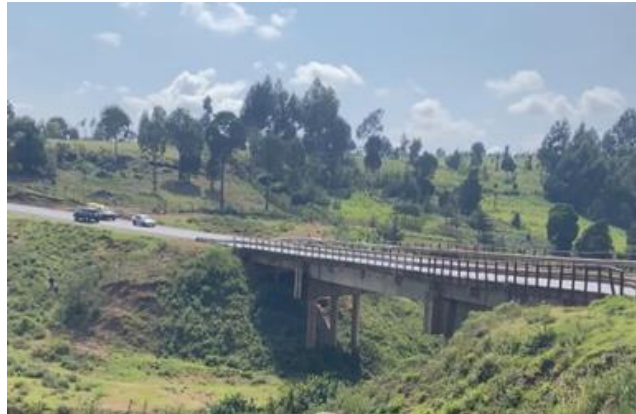
Figure 4: the Sirimon bridge (own photo)
